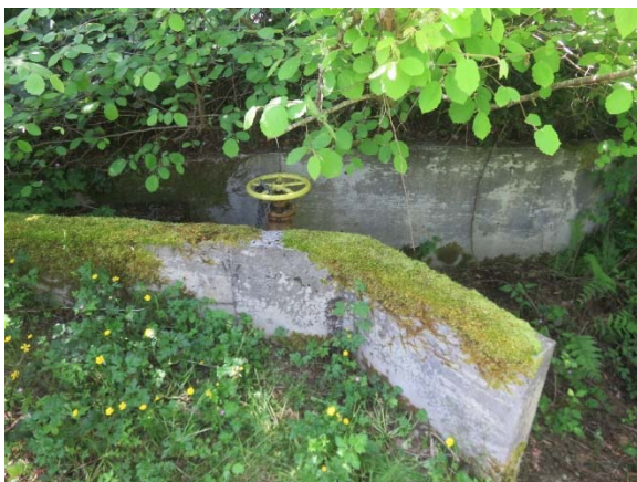
Auxiliary Slide Gate
