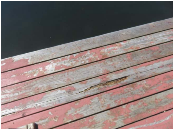
Typical Rot Damage in Decking
