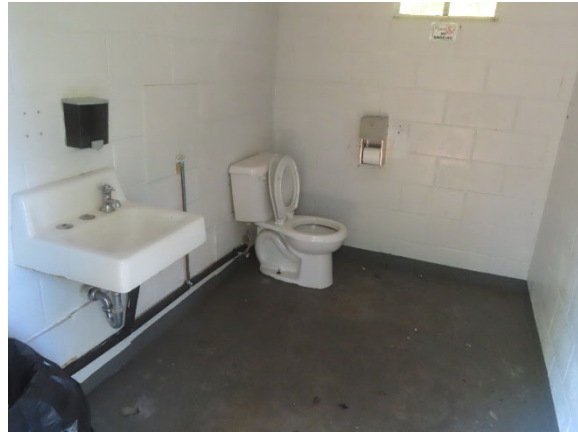
Inside of One of the Two Bathrooms
