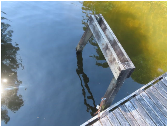
Main Slide Gate
