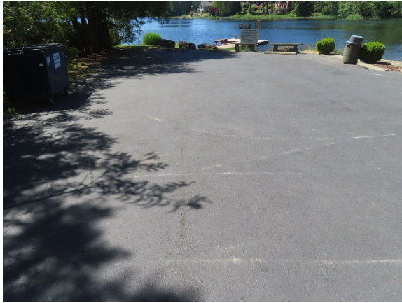
Asphalt Parking Lot at North Beach Area
