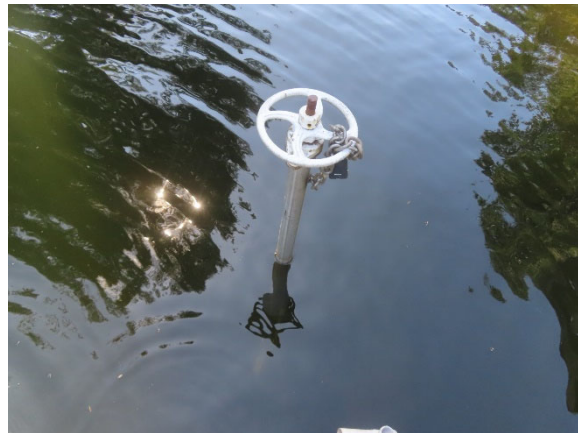
Main Slide Gate
