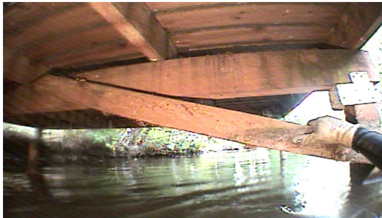
Dock #4 typical underside condition with cross-brace
