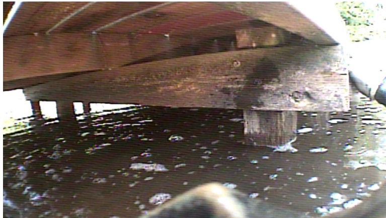
Dock #2 typical underside decking condition
