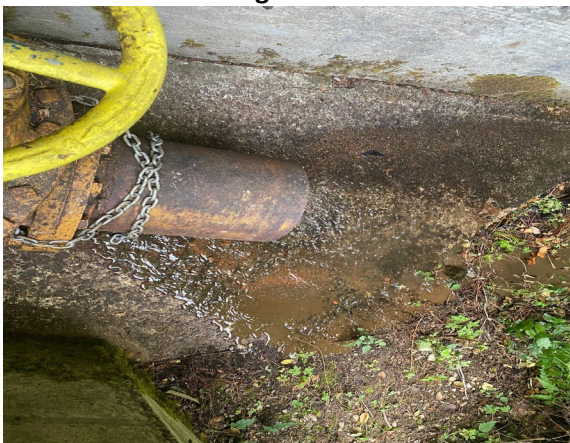
Lower valve flow with upper valve closed
