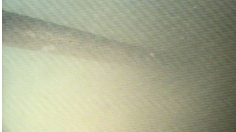
Dock #4 first galvanized steel piling condition
