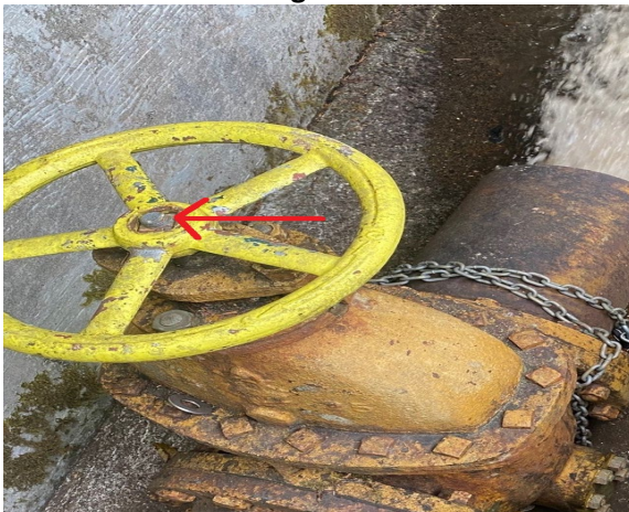
Sheared off threaded valve stem
