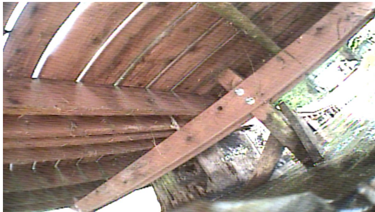
Dock #1 typical underside decking condition
